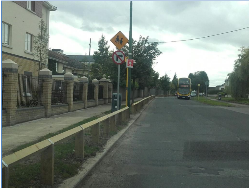
Knee high rails installed on Beneavin Road
